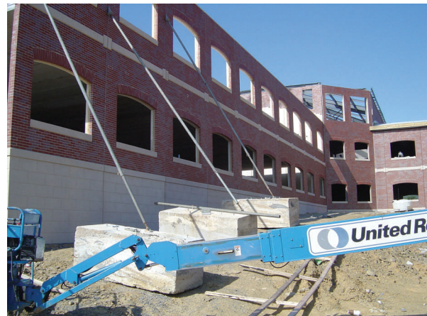
Supplemental support for wall panels while they are set.
