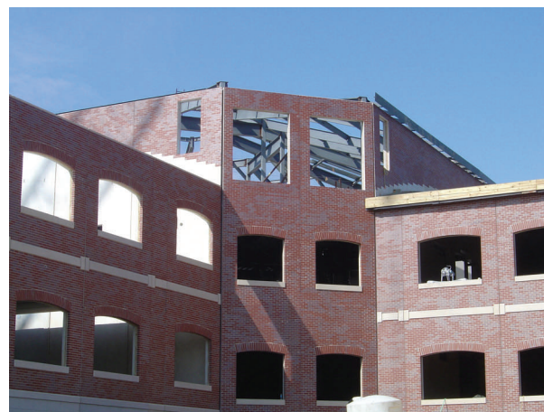
Various wall sections coming together.
