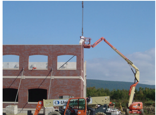
Ensuring proper alignment.
