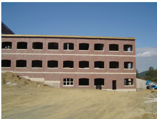
Completed wall section.
