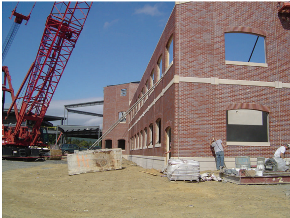
Setting the panel in place.
