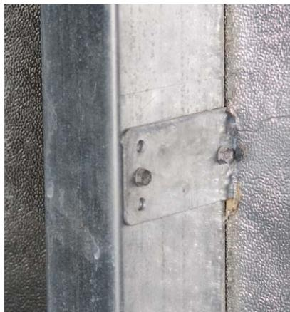
"Look at this – there's no frost on these screws. Typically at this stage only the gypsum would be installed and in this cold (outside temperature: 20°F), you'd really get to see thermal bridging at work: little ice cubes along the stud screws. But THERMAX™ (ci) Exterior Insulation covers the studs and blocks those thermal bridges."
