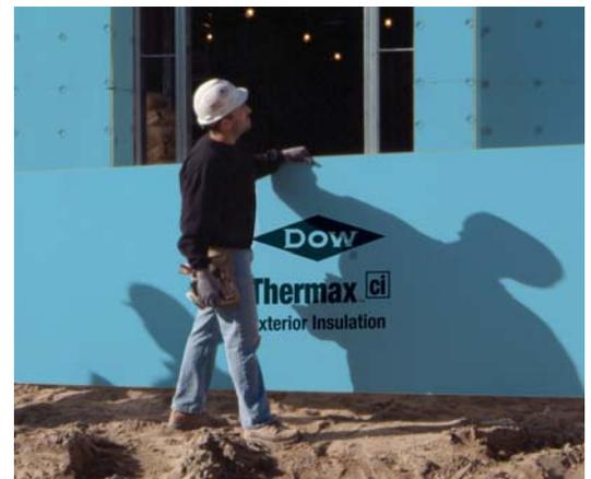
THERMAX™ (ci) Exterior Insulation weighs just 12 pounds per board, compared to exterior gypsum at about 80 pounds per board, allowing faster installation.
