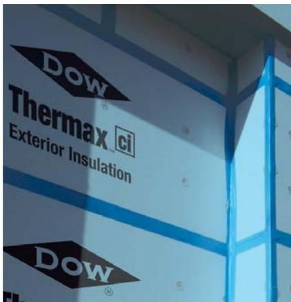
The durable acrylic-coated aluminum facer of THERMAX™ (ci) Exterior Insulation provides a drainage plane and water-resistive barrier, eliminating the extra step of installing a membrane or building wrap. Butyl-based WEATHERMATE™ Flashings protect critical areas against moisture penetration.
