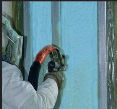
“The THERMAX™ Total Wall System is truly innovative because it reduces the number of trades involved in erecting the wall assembly and, because of the spray-applied interior wall insulation, the smallest penetrations are eliminated.”
